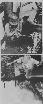
DIVER, aided by hose attendant, drilled underwater bolt holes. BUSADOMI, ayuda dor di base attendant, ta drill buraco bao awa.
